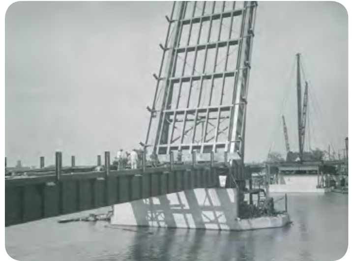
The Lafayette Bridge when constructed in 1938.
