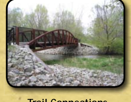
Trail Connections City of Rochester Hills
