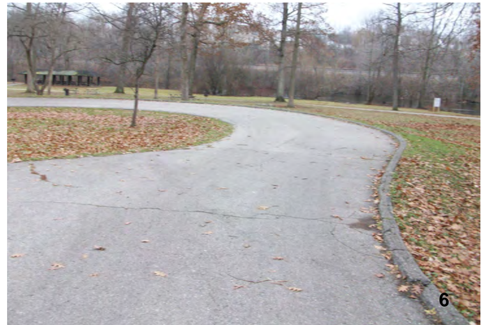
A new aggregate loading and unloading area is proposed along the edge of the turn-around. Some curbing to be removed.
