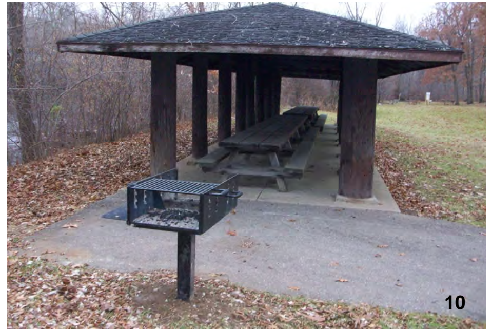
New concrete pavement is proposed under and extending out beyond the roofs edge on all four sides.
