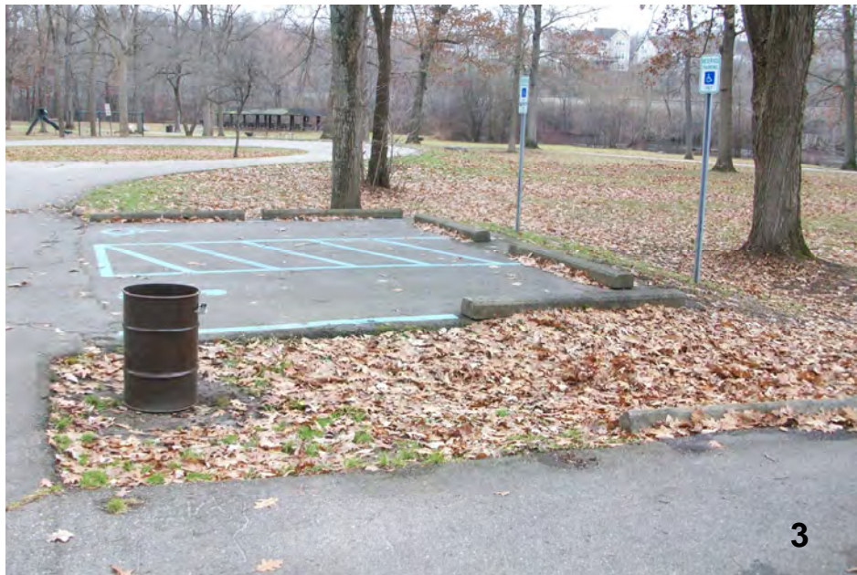
Small turf area between the two parking areas to be filled in with new asphalt. The accessible spaces will be moved slightly so a new universal walk can be constructed to the river and shelter, minimizing tree removals.
