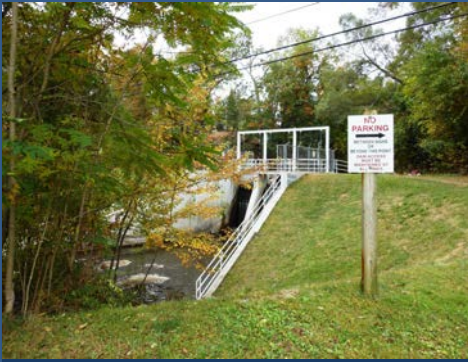
Livingston County Planning Department Hiland Lake Dam
